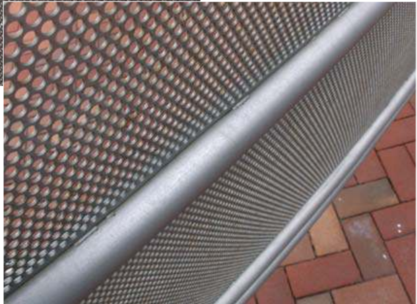
Picture 6. No more rust between the plates and tubes.
