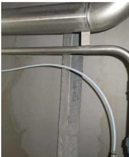
Fig. 2. The rod-shaped magnesium anode is clearly visible in the filter unit of a stainless steel ozone reaction tank (photo by Innomet B.V.).
